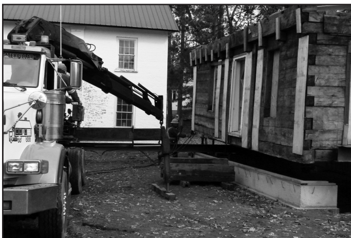
Top: PHK house’s new foundations on the BCHS site.
