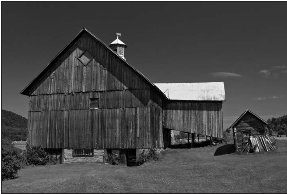
Many high-drive dairy barns were built close to the road to facilitate the pick-up of cream by local creameries. This barn dates from the late nineteenth century and belonged to successive generations of the Jones family in Knowlton's Landing. It has recently been sold for relocation elsewhere in the region. It is typical in its dimensions—forty by sixty feet. A milk house, where raw milk was separated into cream and skim milk, can be seen at right. A horse barn once adjoined the barn, and a wooden-stave silo once stood next to it, too. (Photo: Louise Abbott)
