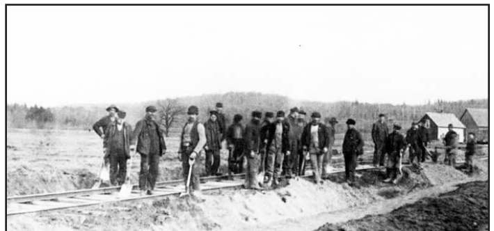
Italian Construction Gang, Orford Mountain Railway, c.1905. Matthew Farfan Collection
