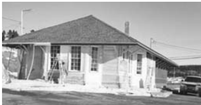
Via Rail spent about $100,000 refurbishing the building, erected during the first decade of the 20th century. The station will again sport its original colours, burgundy, yellow and white.
